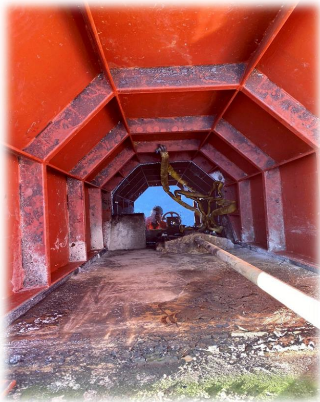
Photo 3: Cofferdam in situ
