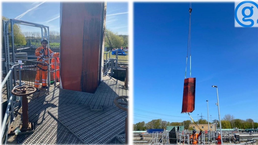
Photo 2: installation of Cofferdams
