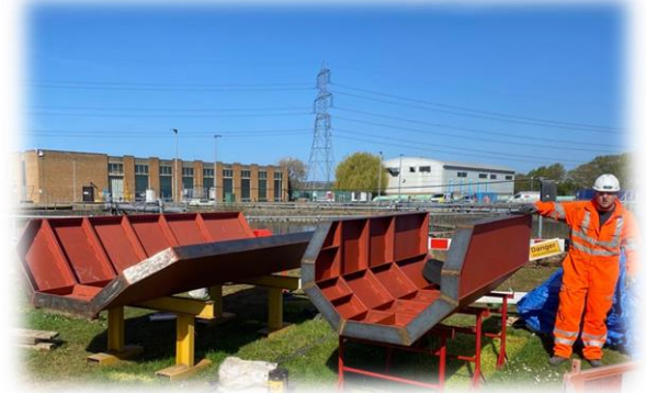
Photo 1: Cofferdams before installation
