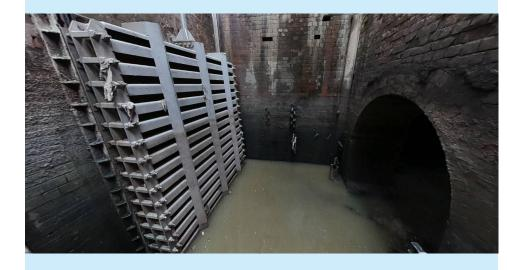
The existing 5no. penstocks at the rear of the Greenwich pumping station were installed in the early 1900's and in a state of disrepair. **GEL** undertook a full 3D model of the wet well to inform the design stage. This allowed the new penstocks to be modelled in such a way that it eliminated any conflict with in-situ assets during the removal and installation processes.
