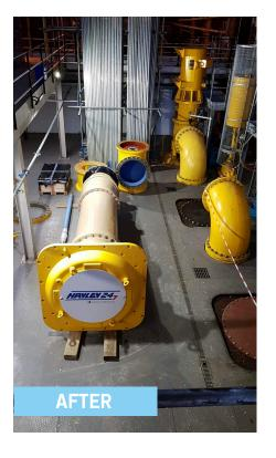
Storm pump no.1 had failed in service with evidence that the pump had run dry causing internal mechanical failures. **GEL's** solution has been to use replace with a completely self-lubricating system with anti-galling and anti-wear. The new innovative seal arrangement pays for itself after 2 years of use.
