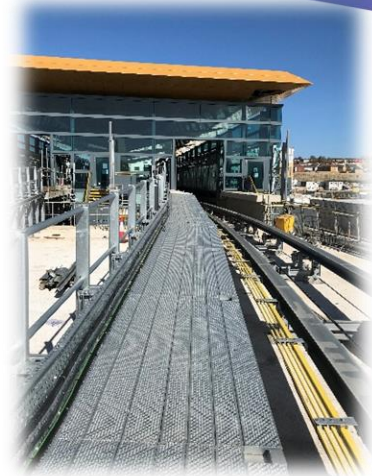
Photo 1: Walkway and guideline entering the terminal building.
