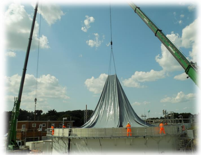
Figure 3 - Attachment of inner membrane
