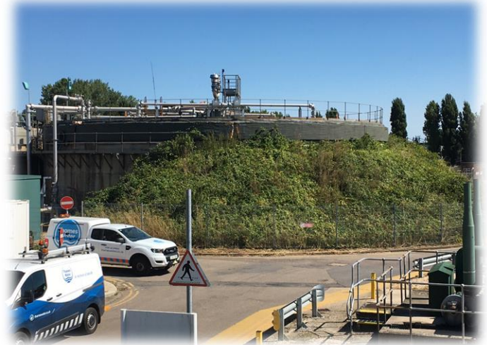
Figure 1 - Digester before start of work.
