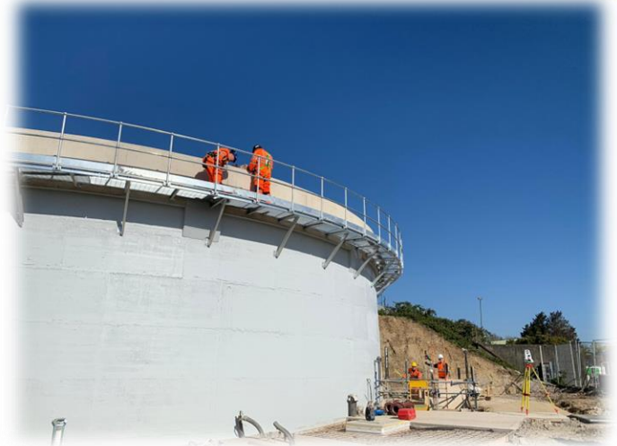
Figure 2 - Upgrade in progress.
