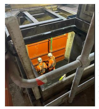
• **GEL** was asked to design, fabricate, and install a Temporary and a new stainless steel stop log frame and stop logs for future use to the existing inlet channels serving screens 4a & 4b, to allow secondary isolations to the inlet channels. They will also be utilised for future use on screen channels 1a, 1b, 3a, 3b, 5a & 5b.
